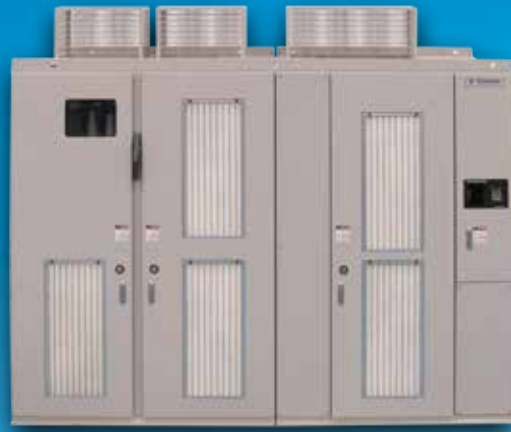
MV1000 Drive: 2000 HP, 4.16 kV, with Input Switchgear
