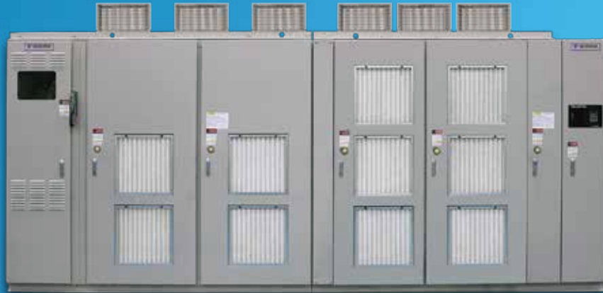
MV1000 Drive: 3000 HP, 4.16 kV, with Input Switchgear
