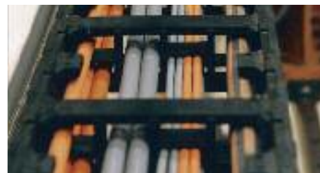
Neatly laid cables with iglus® interior separation
