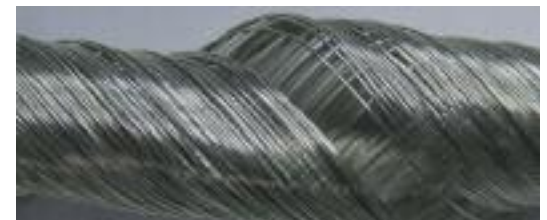
Detailed analysis of the tested CFROBOT cable show no damage. See picture above.
