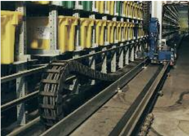
Automated storage/retrieval system with System E2 and Chainflex® cables - travels up to 262 ft (80 m) and speed of 14.8 ft/s (4.5 m/s)
