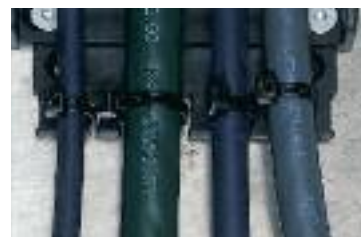
Simple strain relief with cable tiwraps attached to igus® tiwraps plates and integrated into the mounting bracket
