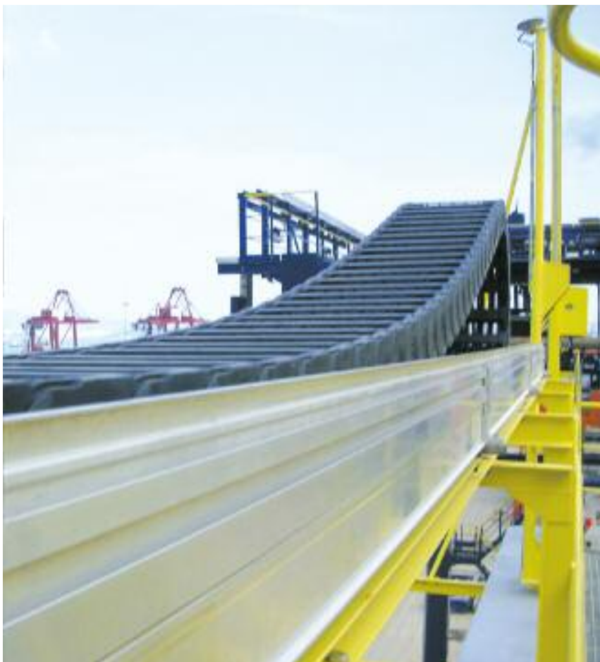
Seawater resistant aluminum “SuperTrough” in a RTG-crane. Long travel with the E4/4 Energy Chain System®.
