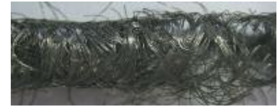
Samples of the cable were cut and analyzed at sections along the tested cables length. In the image above damage of the overall shield are noticeable.
